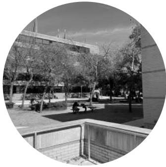
Existing Retaining Wall
