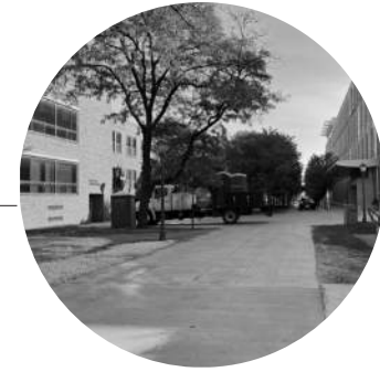
Existing Straz Hall
