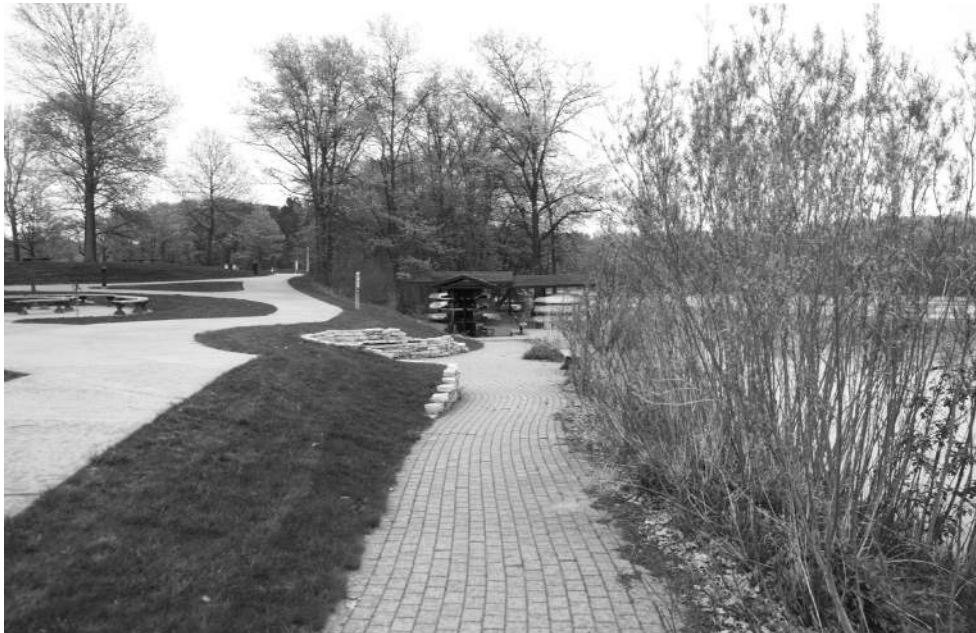
Existing accessible walk was in disrepair and shoreline was overgrown.
