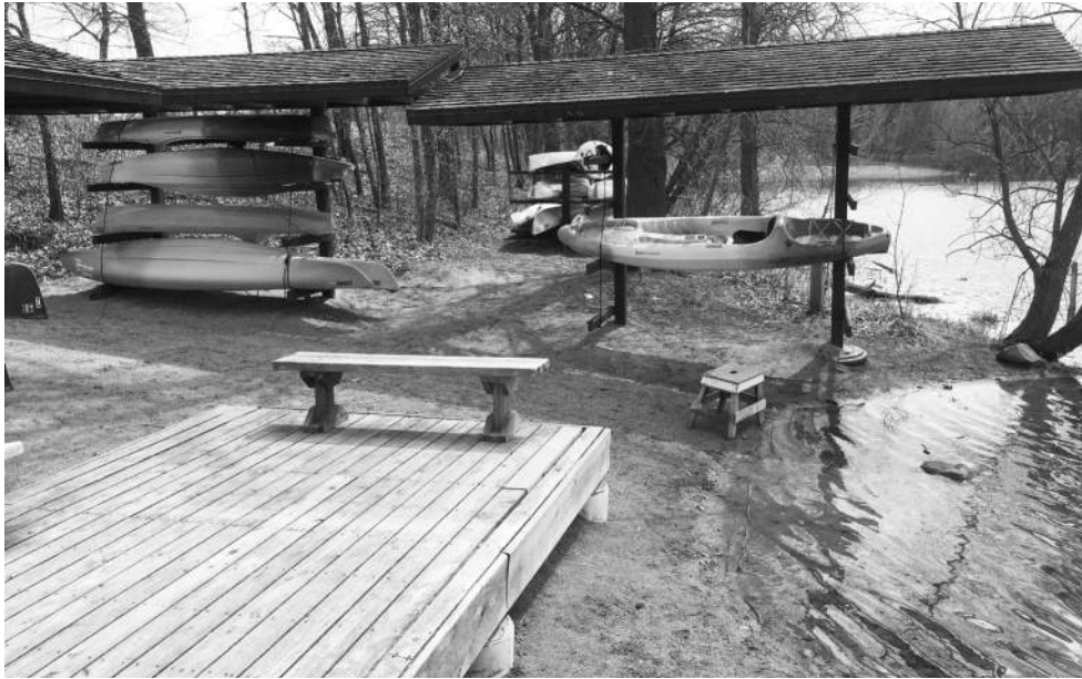
Storage racks were difficult for staff to use and water access was not accessible.
