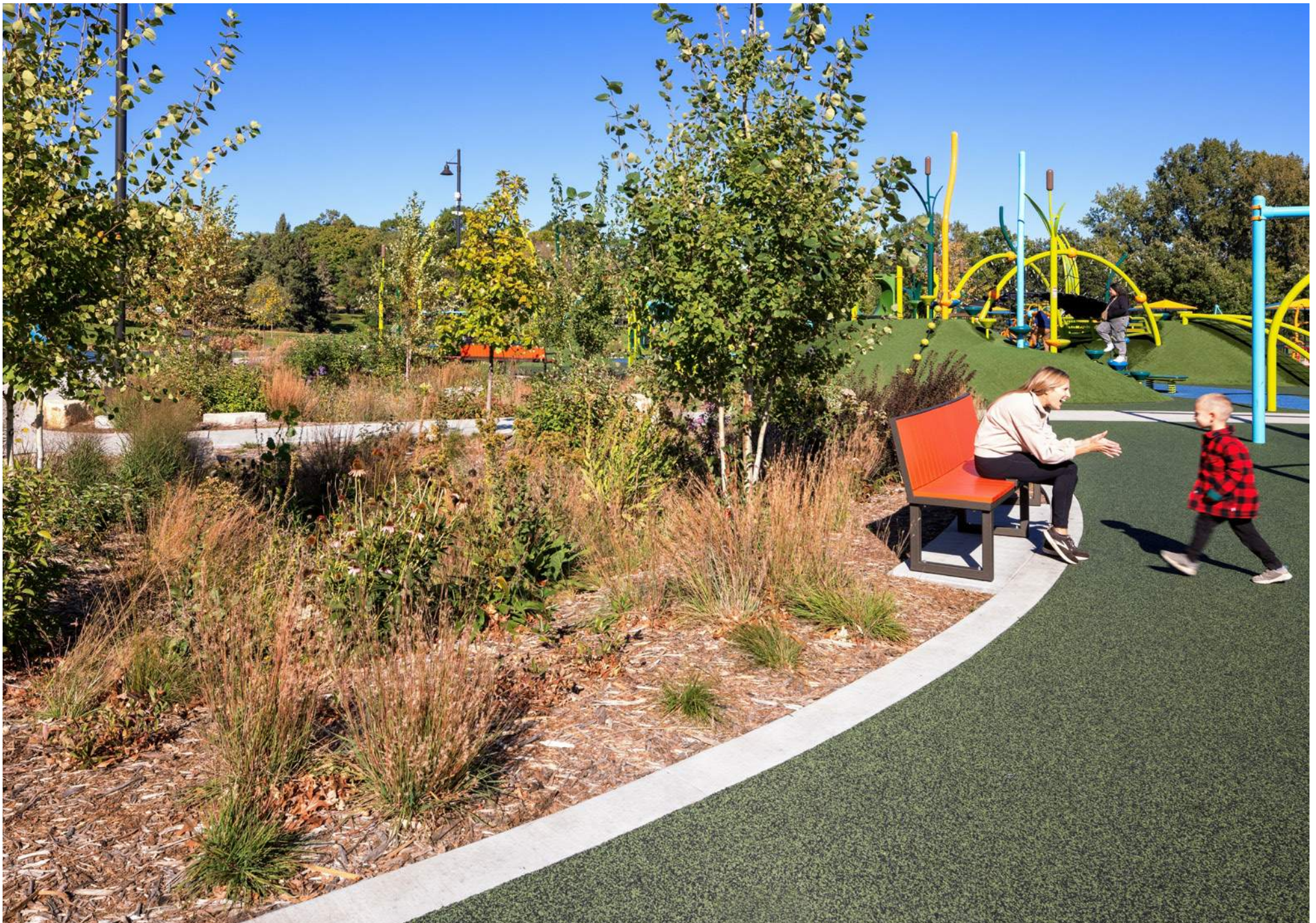
Interconnected raingardens and biofiltration basins manage stormwater for the destination playground and were used to define distinct play experiences and gathering areas.
