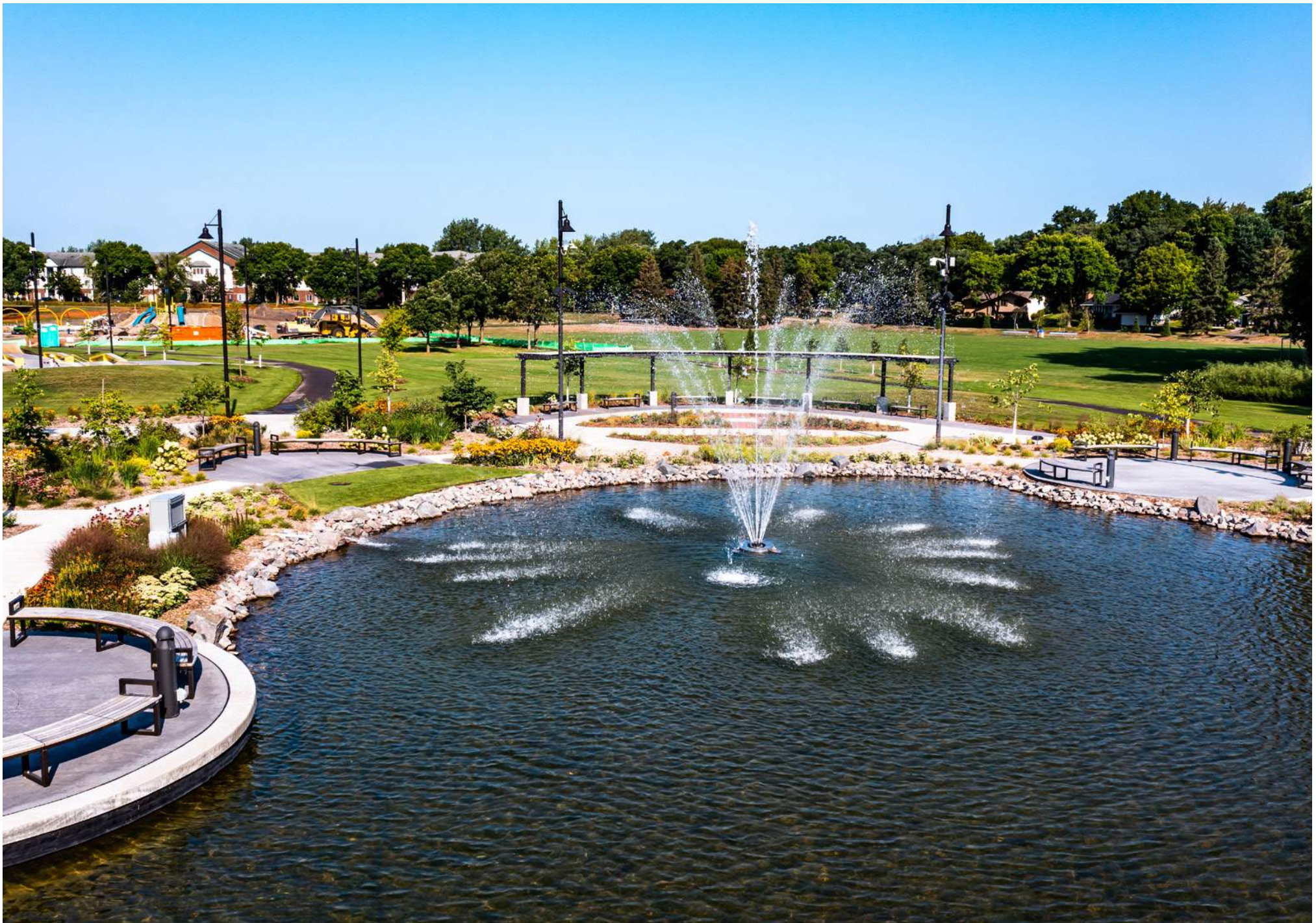
The central fountain feature is a key part of the stormwater management system, reusing water to irrigate the gardens and a large portion of the park. In this image, Phase 1 is complete in the foreground and Phase 2 is under construction in the background.
