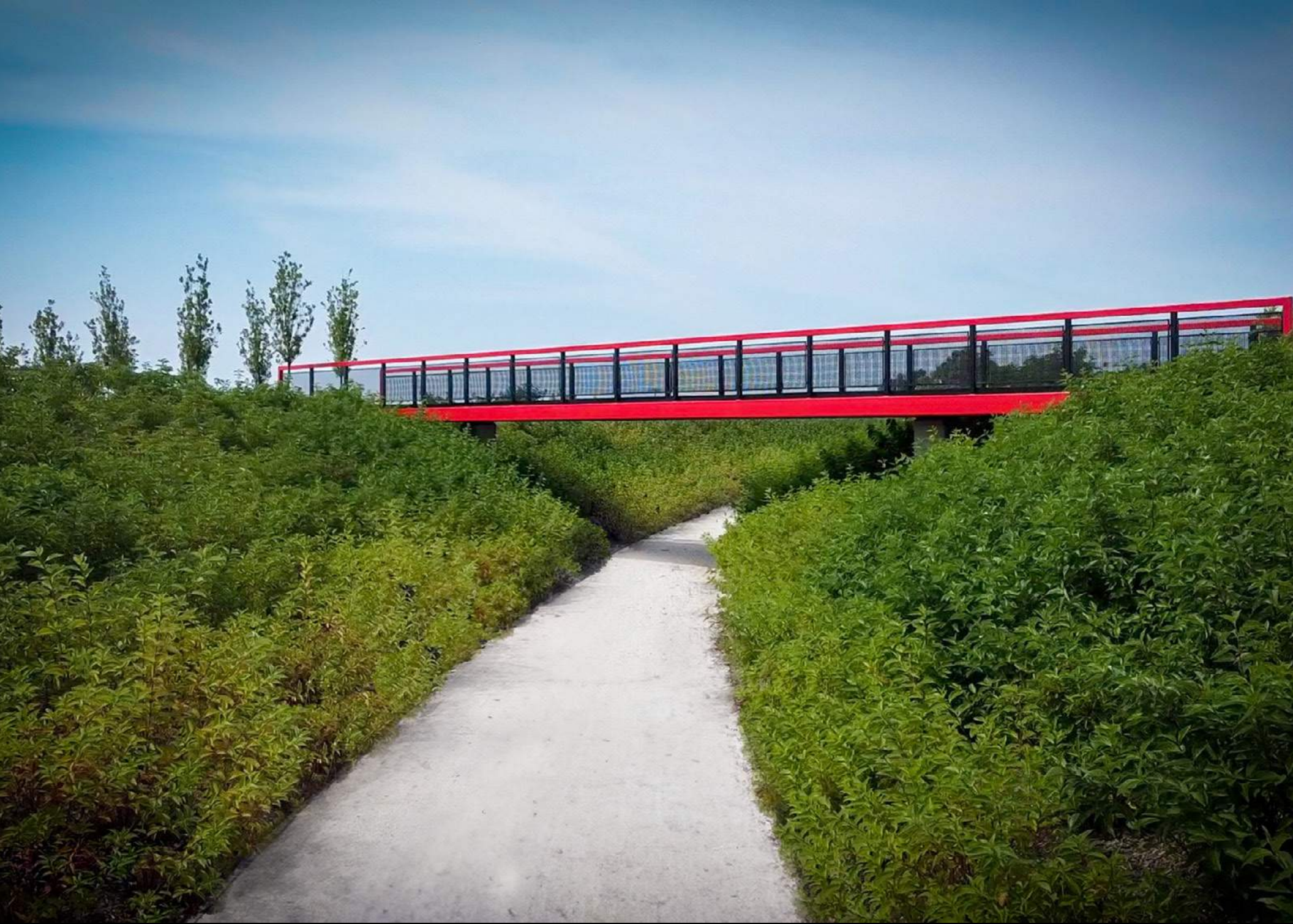
The rampart features densely planted slopes with bridges across the top. The design is inspired by trench warfare. Visitors can walk the mile-long trail, experiencing shifting perspectives from enclosures to openness.
