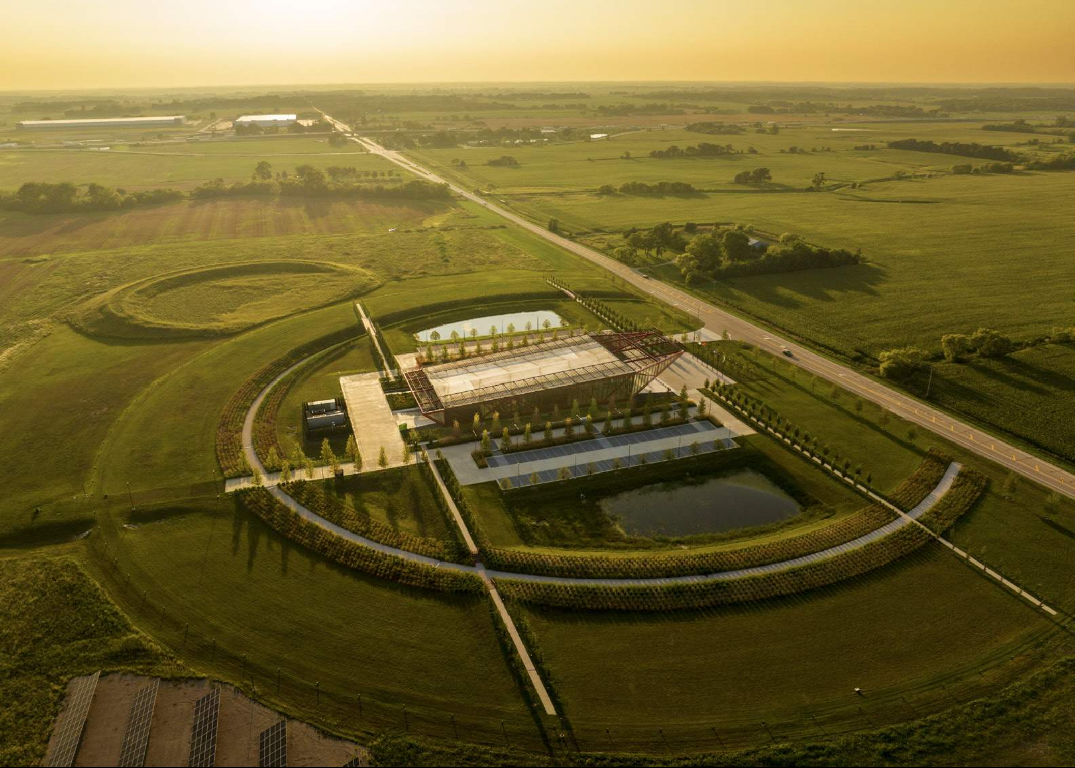
Bird's eye view of the completed project under dusk
